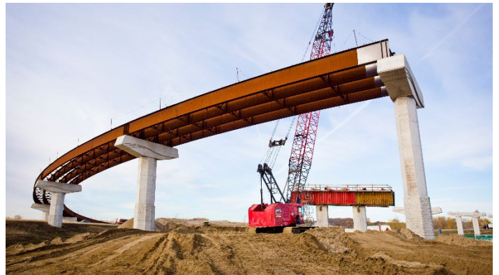
I-80 and I-29 interchange construction
