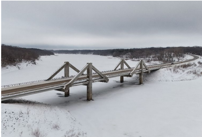
Mehaffey Bridge near Solon
