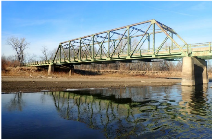
Steel Thru Truss
